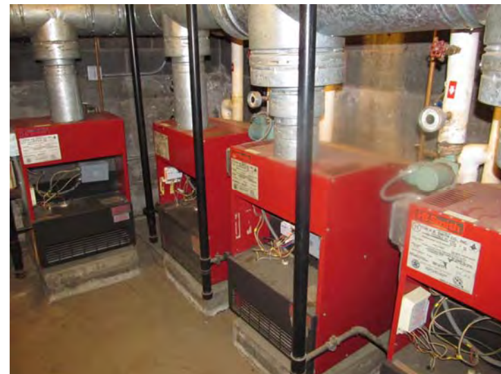
HB Smith boilers for production of hydronic heat.
