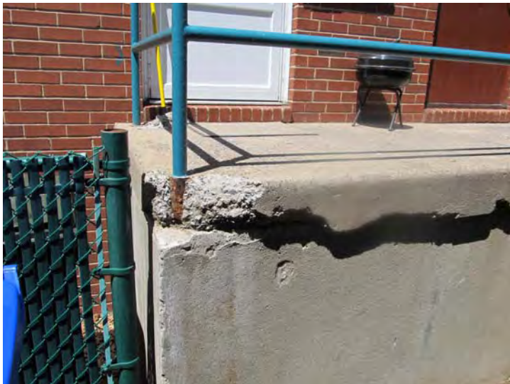
Areas of spalled concrete noted at the concrete stoops.
