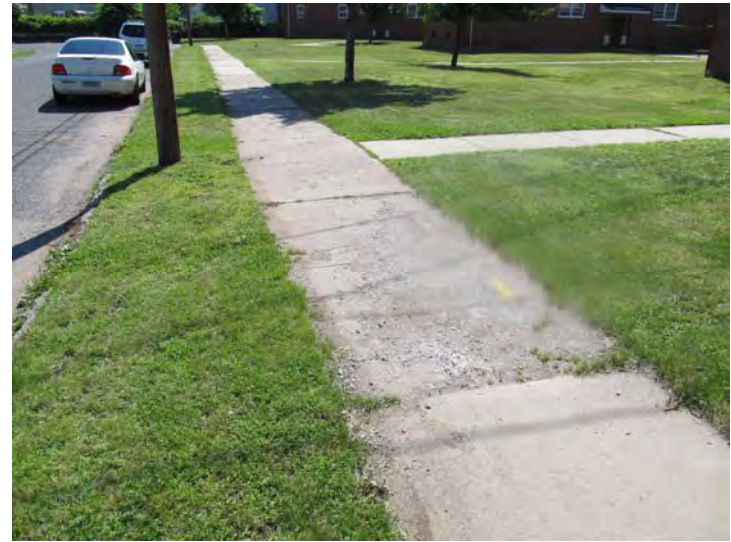
Areas of cracking and surface scaling noted at the concrete sidewalks.
