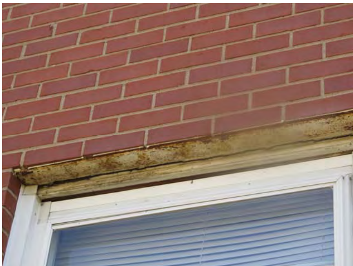
View of surface corrosion on steel lintel.
