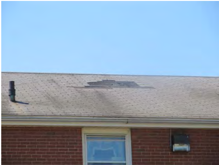
View of missing and deteriorated composite asphalt shingles.
