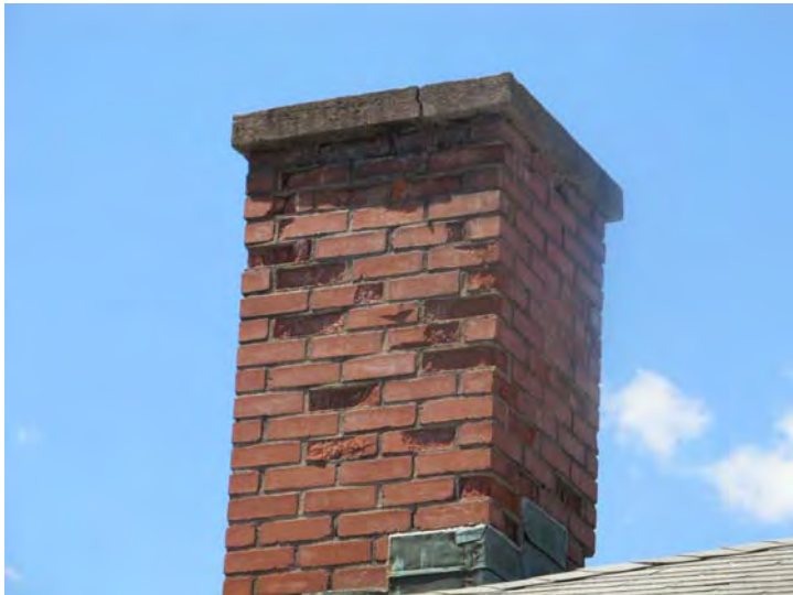
Spalled brick noted at chimney – Maintenance building shown here.
