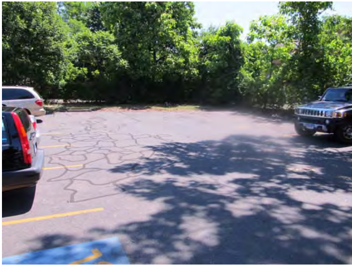
View of crack seal repairs to the asphalt paved surfaces.
