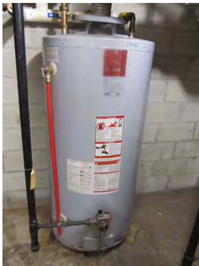
State Select gas fired hot water heater.
