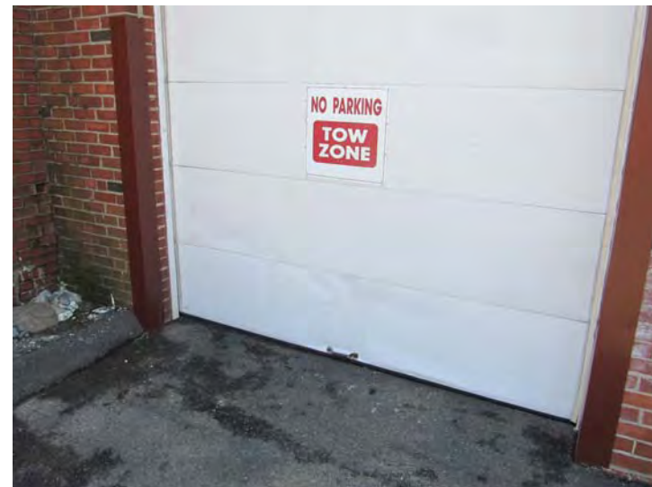
View of metal overhead door exhibiting impact damage at maintenance building.
