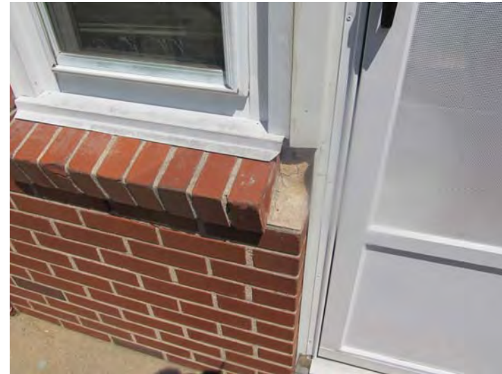
Missing brick masonry unit noted at rowlock window sill.
